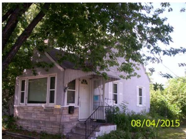
South and east sides, posting
