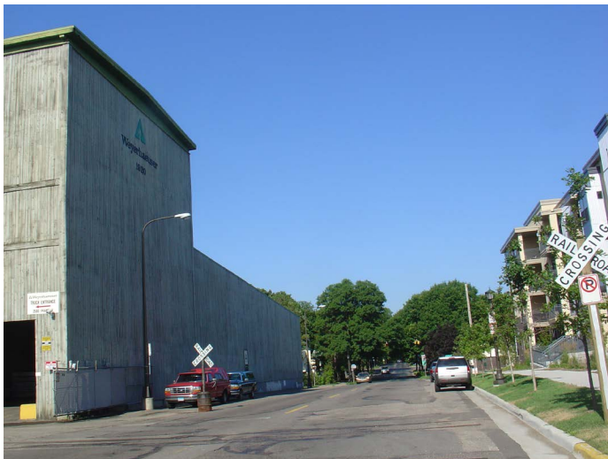
Residential/industrial interface on Franklin Avenue and Berry Street
