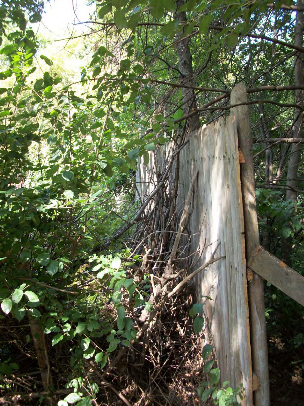
8 West section looking West from the middle section
