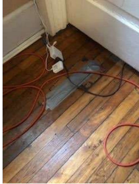
33: Tape to repair flooring in tenant unit
