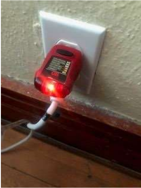
43: Testing unit showing open ground outlet
