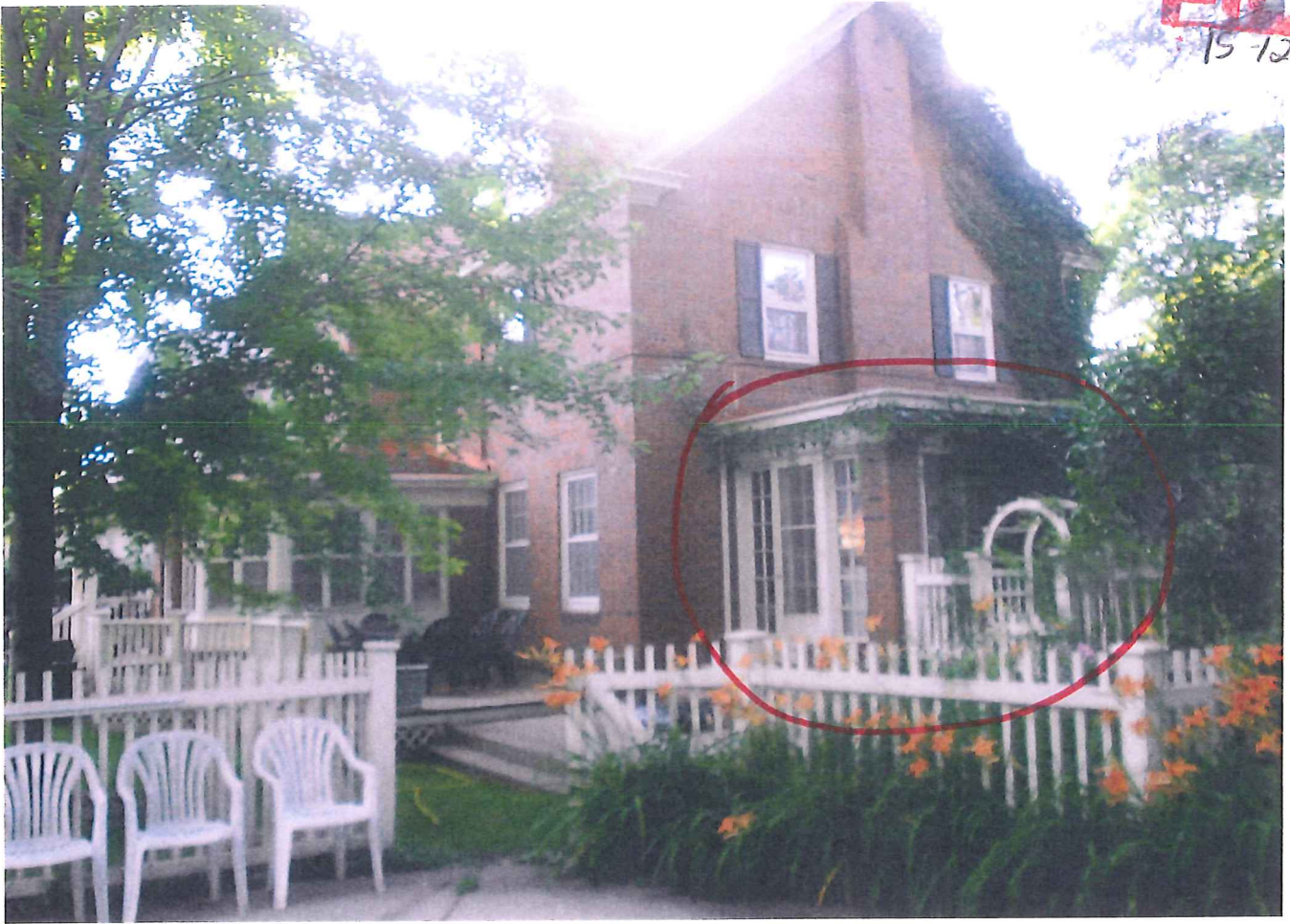
REAR AND SIDE VIEW OF THE HOUSE'S SUNROOM. STANDING IN THE SOUTH LOOKING NORTHWEST.
