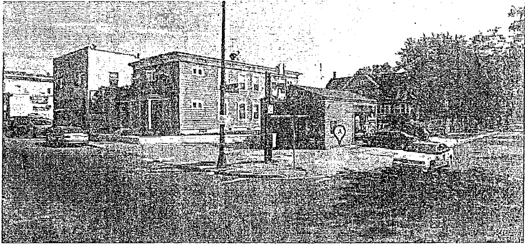
Fig. 1. View of 902 Arcade St & 908 Arcade St, looking northeast from York/Arcade intersection
