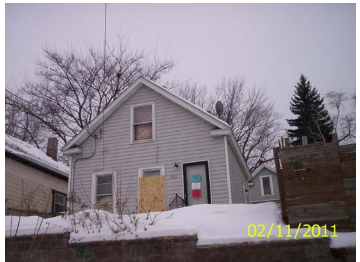
East and north sides, posting
