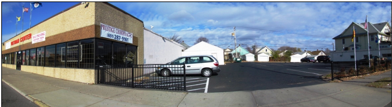
The Vietnam Center at 1159 University Avenue.
