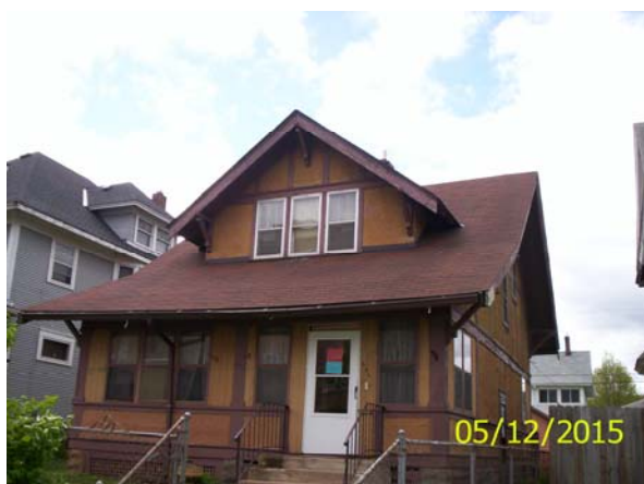
North and west sides, posting
