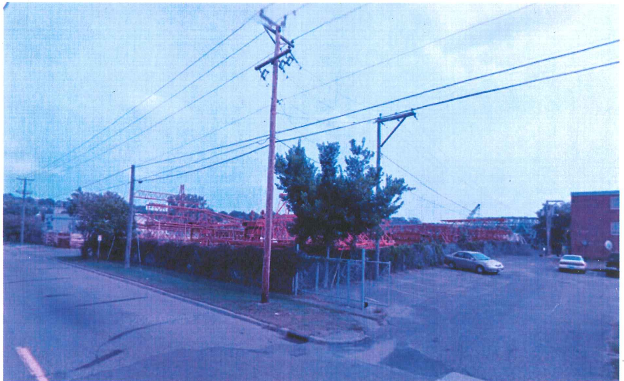
Fig. 2. Northeast view of property line between 1394 Jackson St & neighboring property to the north (Advance Shoring)
