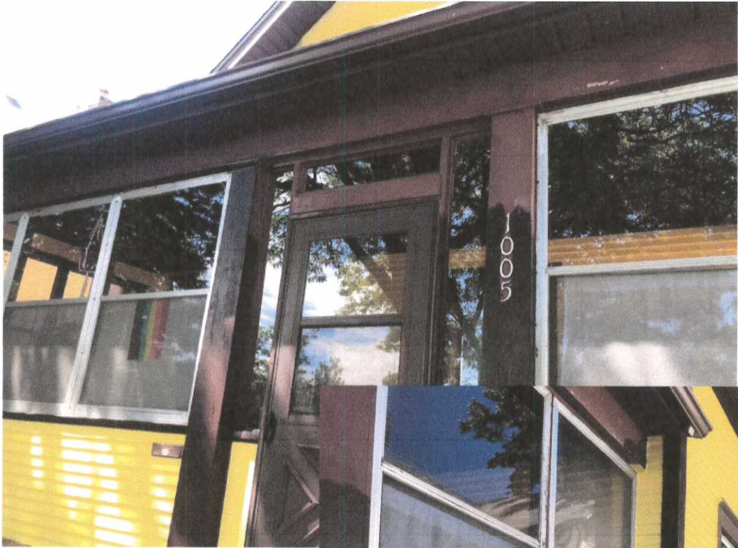
Photos from Contractor 6/21/22
