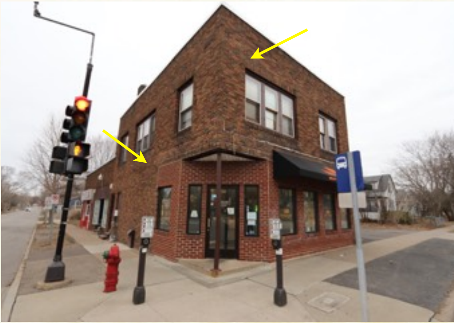
These two elevations were reviewed for masonry restoration needs.
