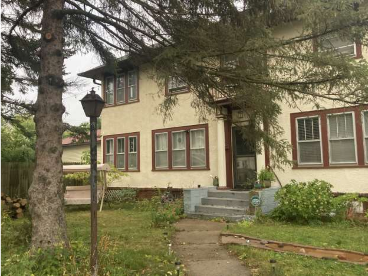
957 Flandrau St.Owner Photos.6-19-24
