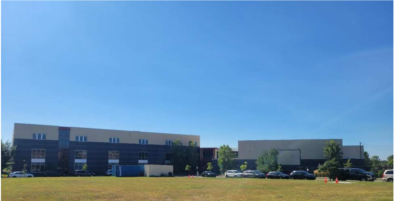
Nova Classical Academy along Mercer Way and Madson Street.; image taken from the subject parcel.
