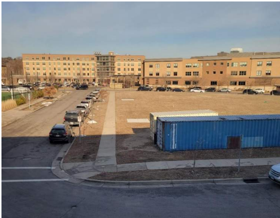
Shalom Campus and the subject parcel from the corner of Madson Way and Mercer Street.
