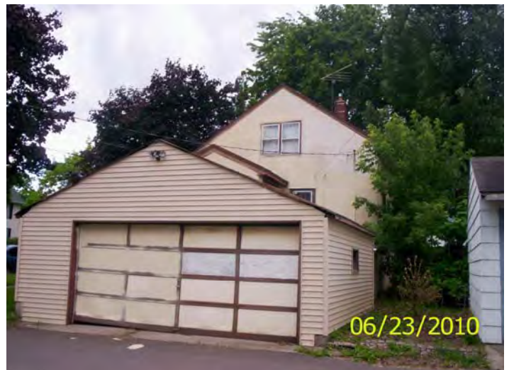
Garage, north and west sides
