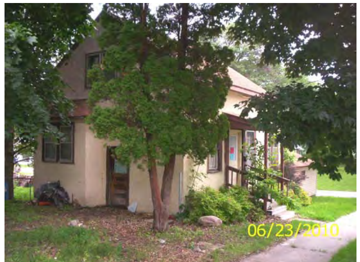
South and east sides, posting
