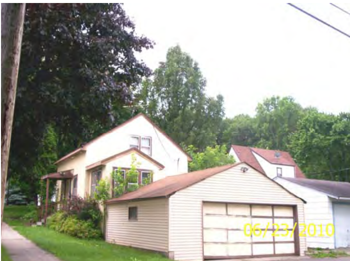
East and north sides, garage
