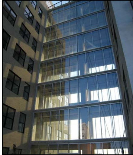
Figure 3.2.2.5.1: Example of fully glazed passageway
