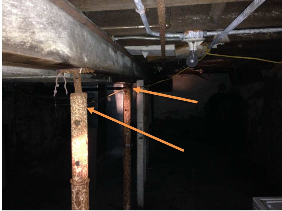
Picture 9 – Shoring Columns Supporting a Beam
