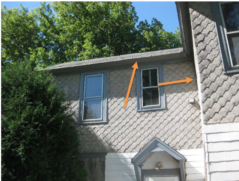
Picture 14 – House Roof and Exterior Wall
