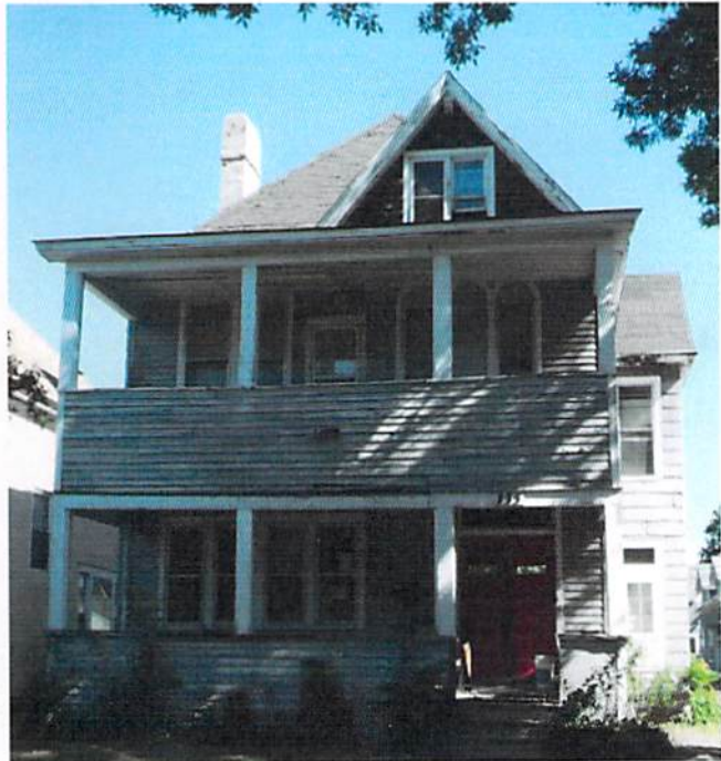
FRONT STREET VIEW –JUNE 2018 735 MARGARET STREET ST YEAR BUILT: 1890
