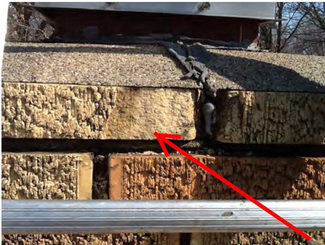
Cracks in wash at the top of the chimney
