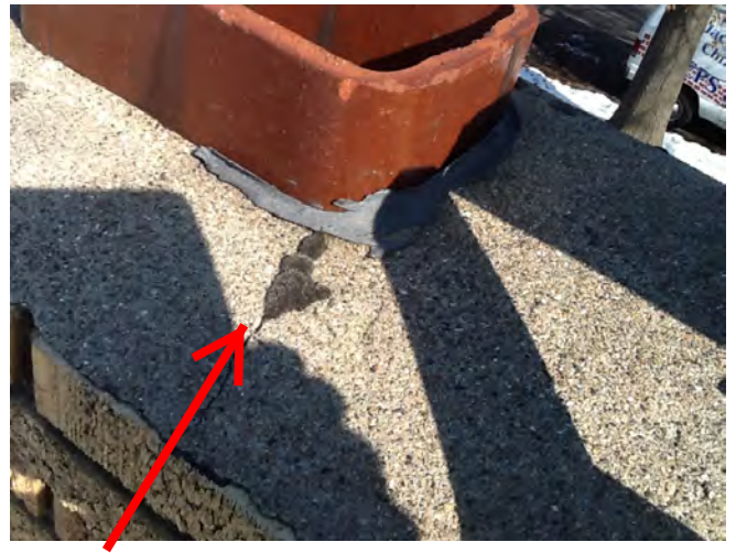
Cracks in wash at the top of the chimney
