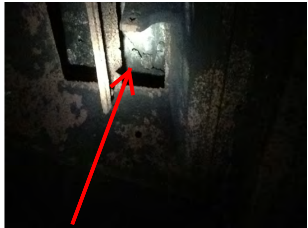
Wood in lintel area of the lower level fireplace
