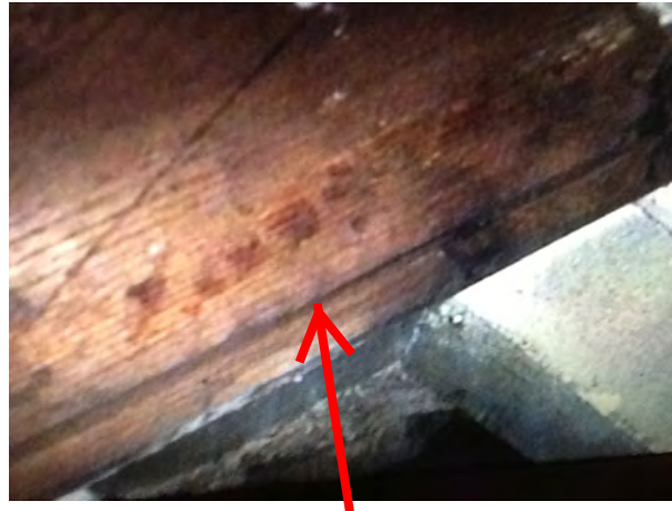
Wood in ash dump of main level fireplace
