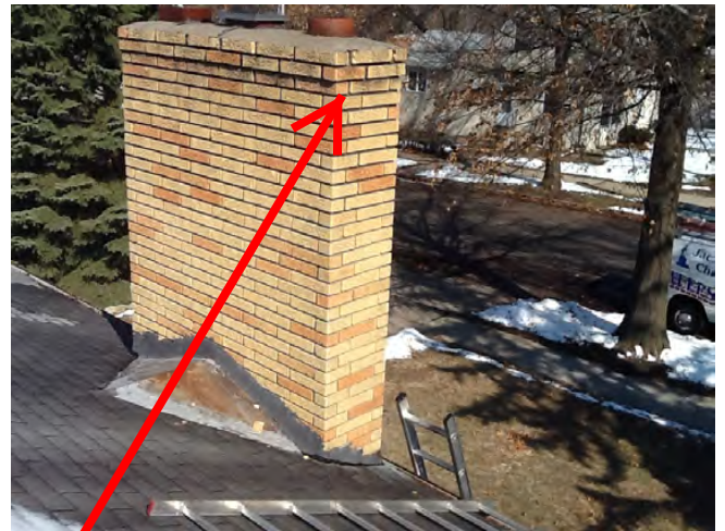
Spalling brick and deteriorating mortar joints
