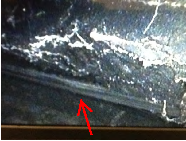
Wood in lintel area main level fireplace
