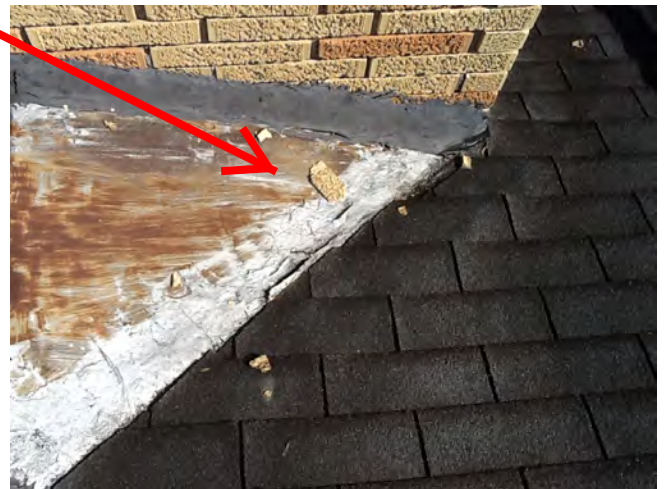
Spalling brick and deteriorating mortar joints
