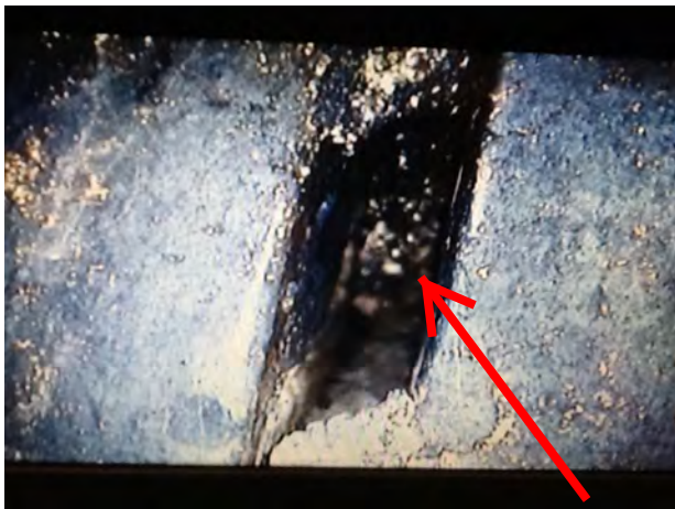
Gaps around the bricks and the bottom flue tile in main level smoke chamber
