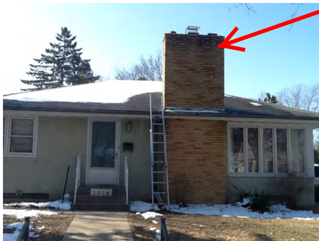
Spalling brick and deteriorating mortar joints
