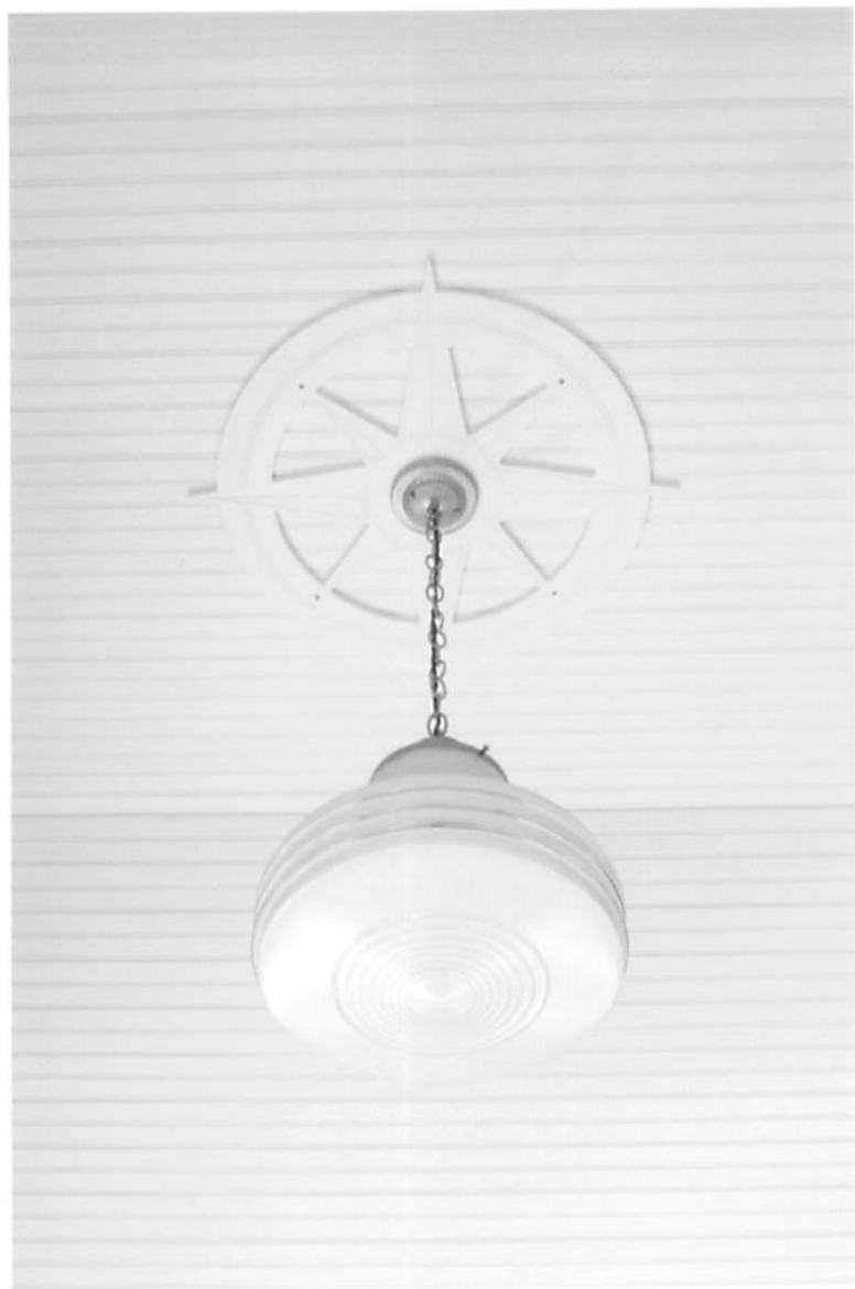
New Porch Ceiling 2015
