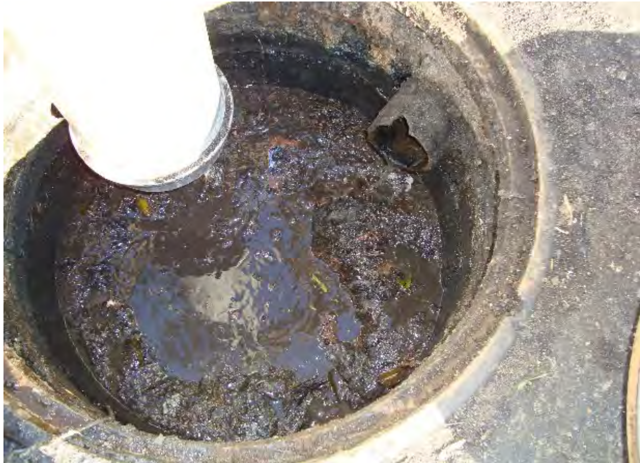
Sanitary Discharge, Private Storm Drain
