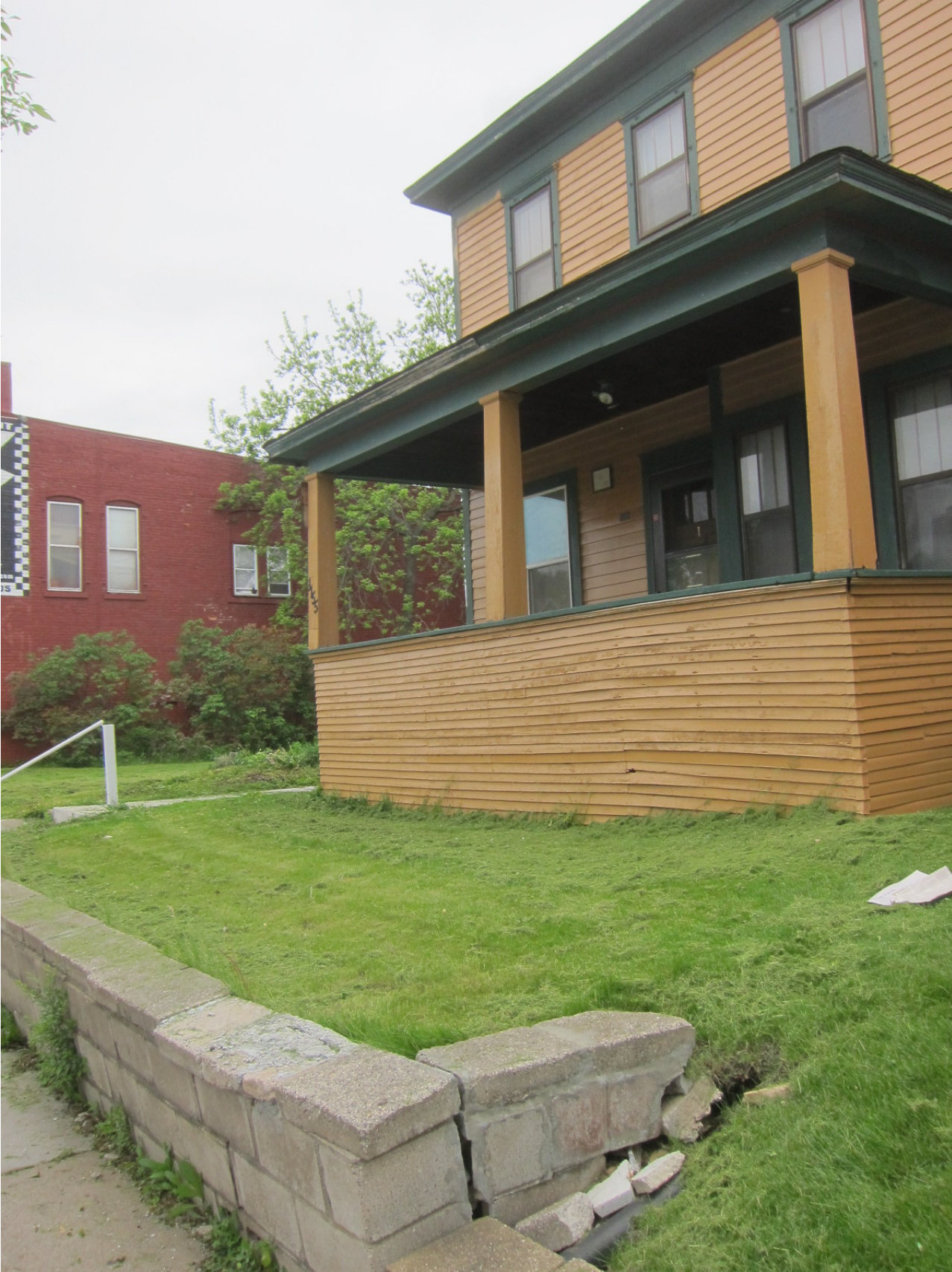
Front of building – deteriorated and leaning retaining wall
