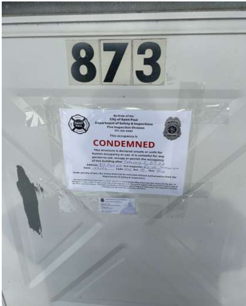
873 Front Ave. Condemned Placard
