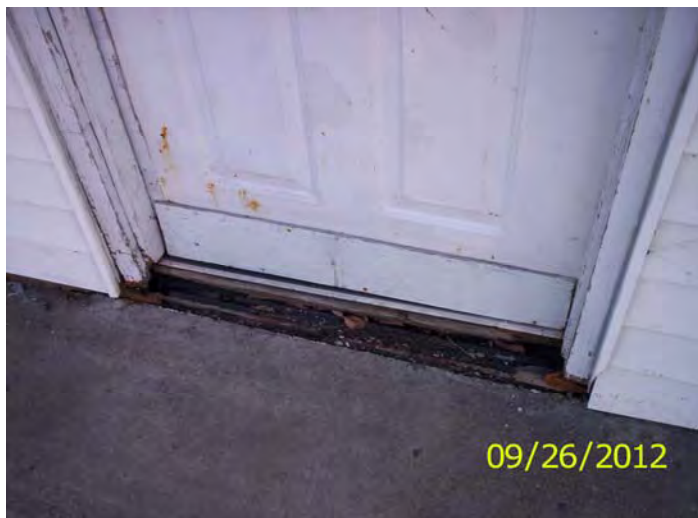
Front door threshold
