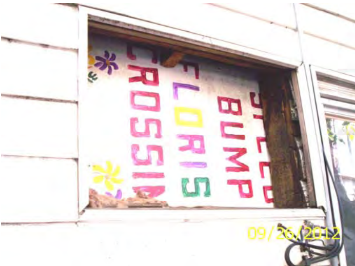
Opening in the north wall
