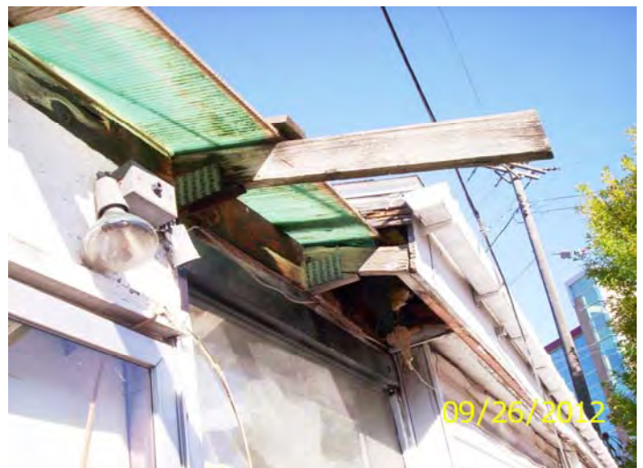
South side eave
