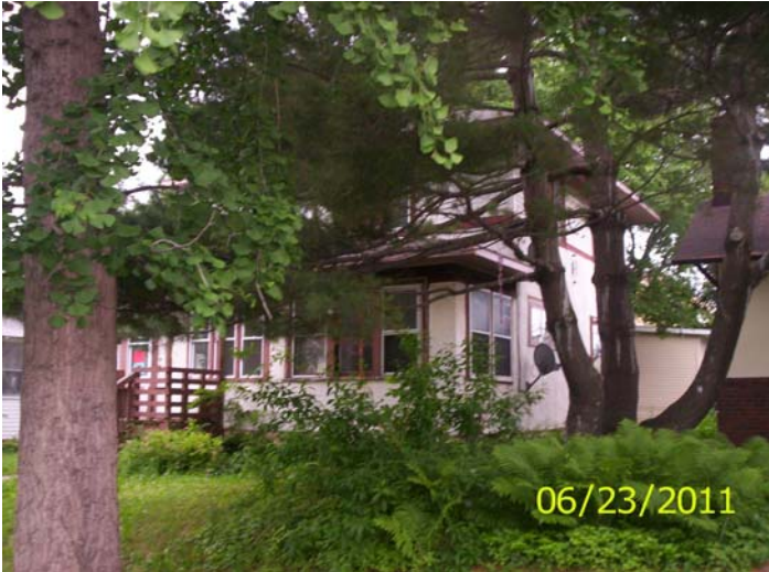
North and west sides, posting
