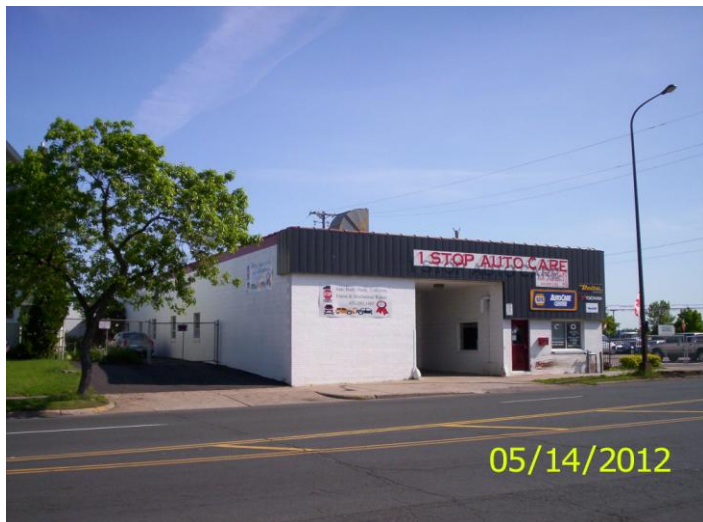
Front view of bldg secured
