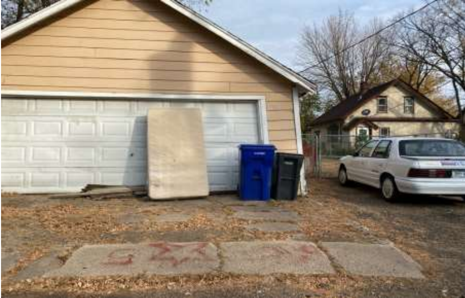
864 Case Ave.Photos taken when reinspected on 11-5-24
