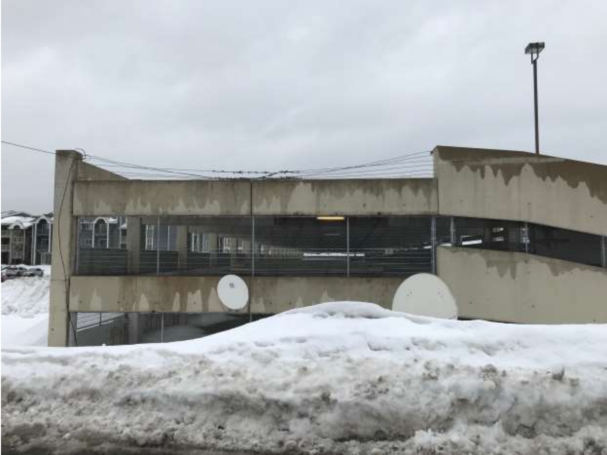
1015 Bandana Blvd W. Photos 3-1-23
