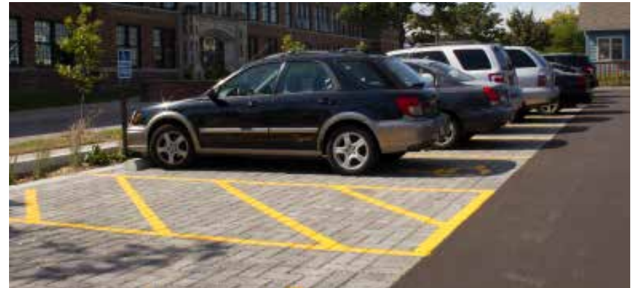
Example of a permeable pavements
