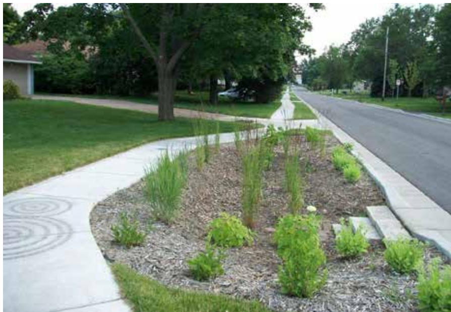
Example of vegetated swale in Maplewood
