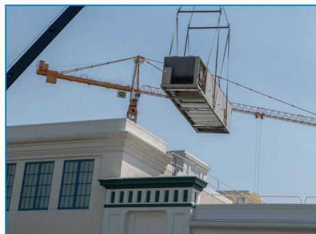
A new heating, ventilation, and air conditioning system was installed at the treatment plant on Friday, August 4.
