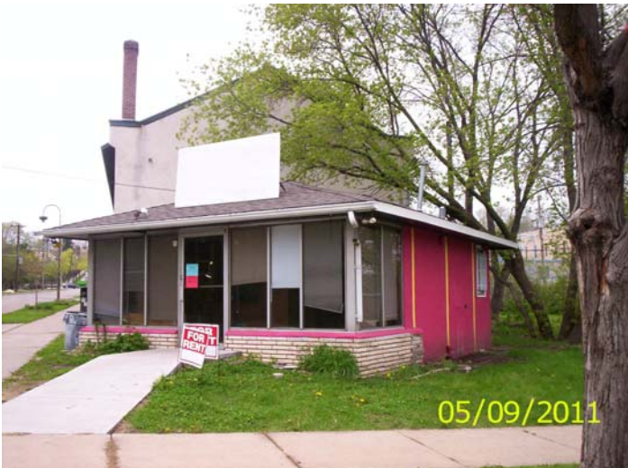
East and north sides, posting
