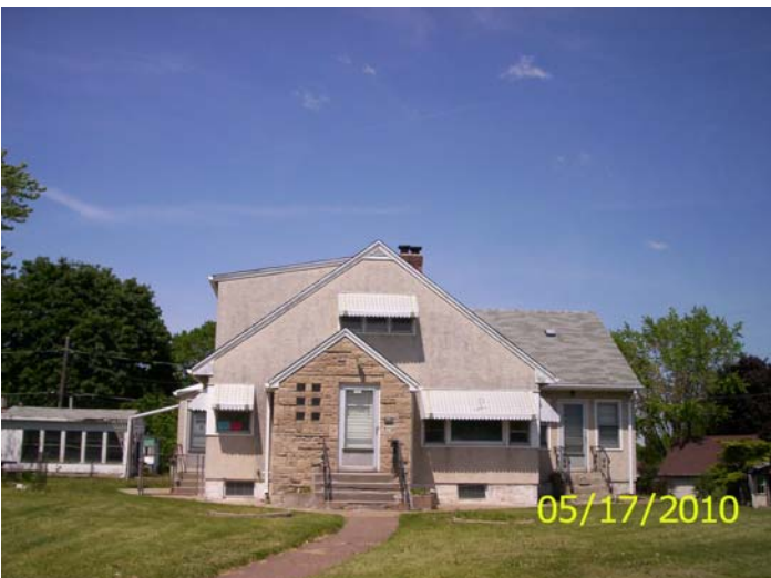
South side, posting
