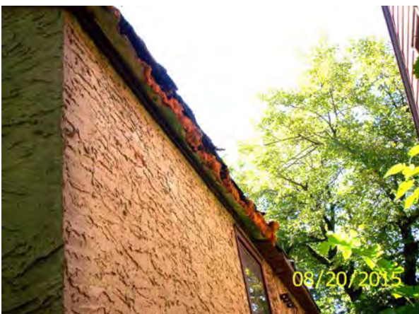
West side eave
