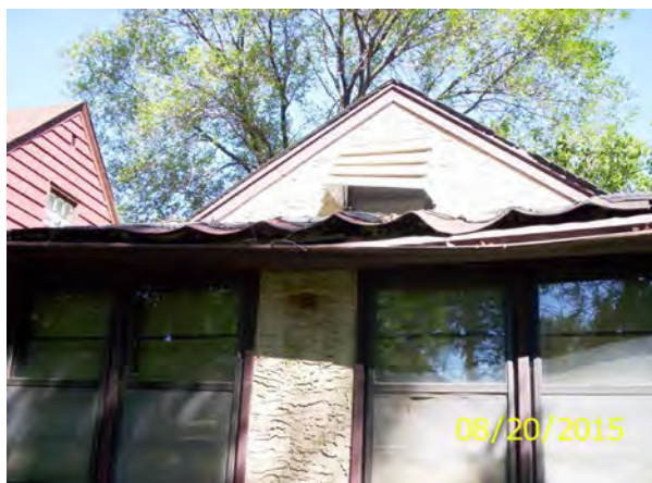
South side eave
