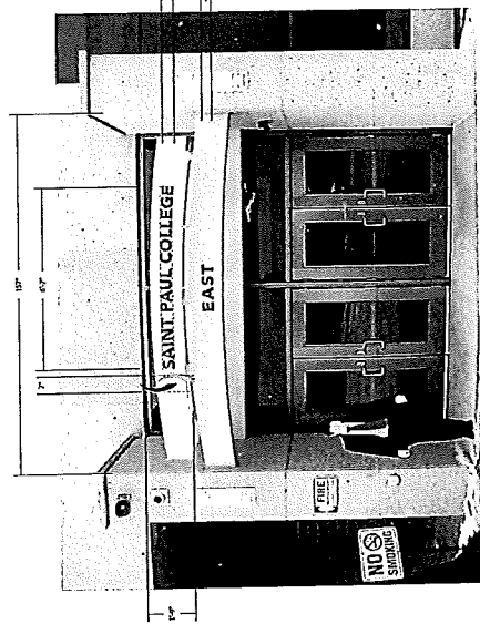
4 OPTION 1 - EAST ENTRY - INDY, NON LUMI, DARK BLUE LETTERS (PANTONE 280, PMS 281) ON EXISTING LIGHT GRAY CURVED ALUM. PANKS 1\"/>
