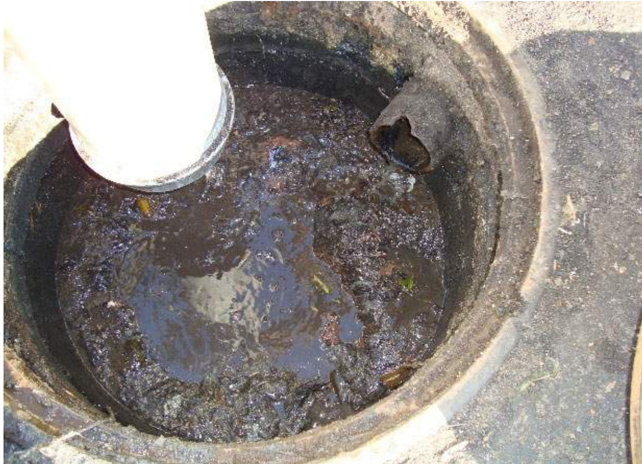
Sanitary Discharge, Private Storm Drain
