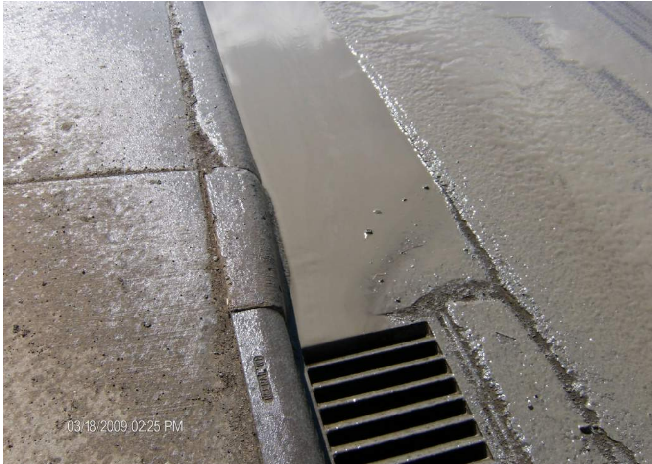
Discharge of Drilling Mud
