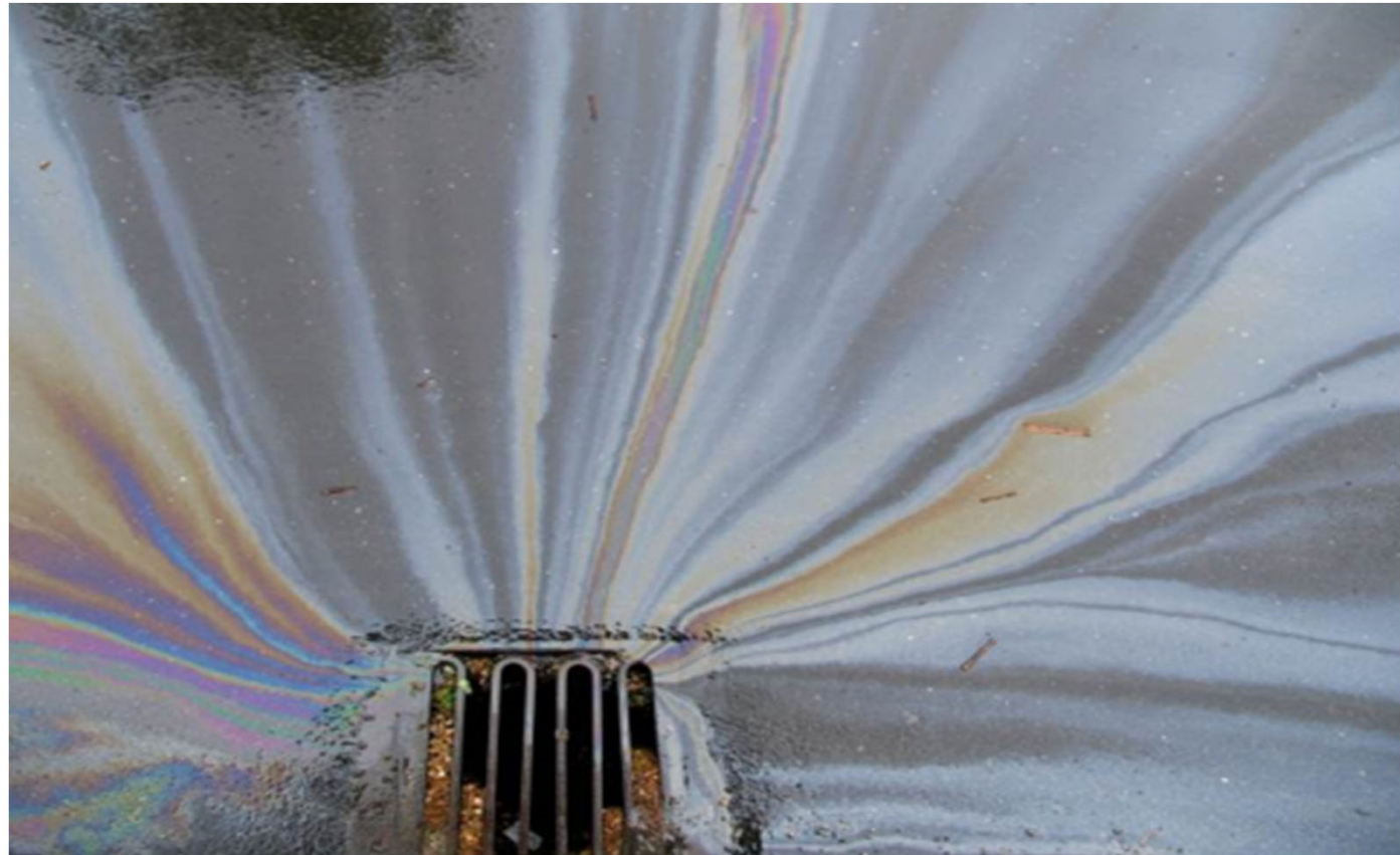
Discharge of Oil
