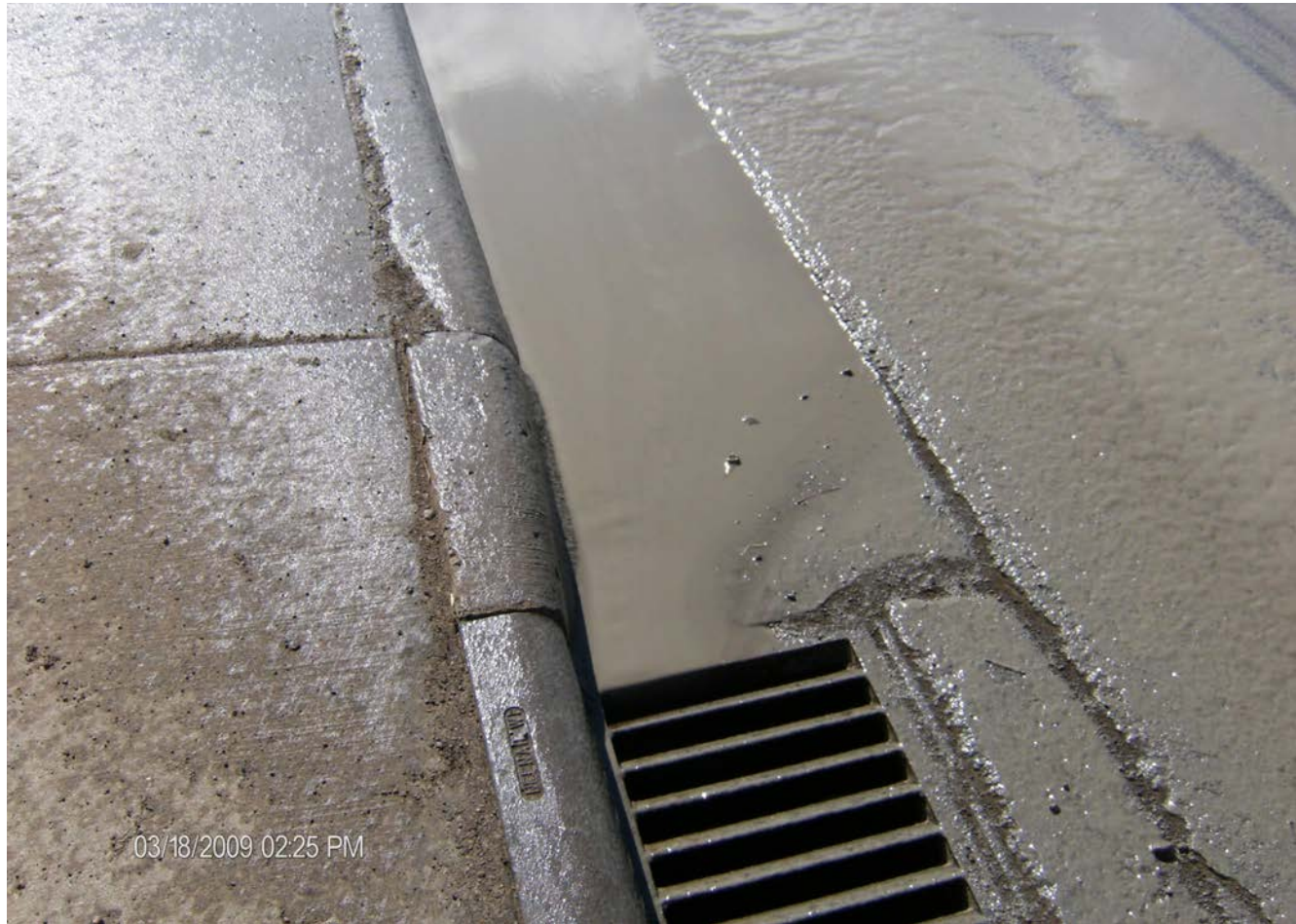
Discharge of Drilling Mud
