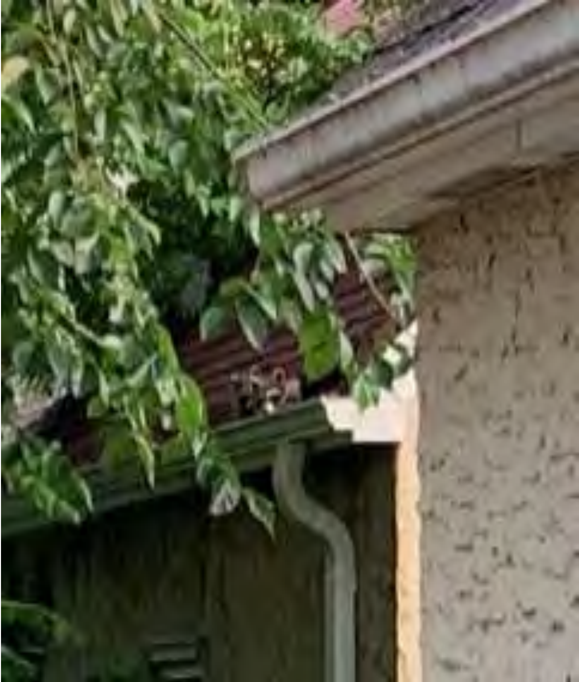
1372 Victoria Ave -Neighbor took these photos
