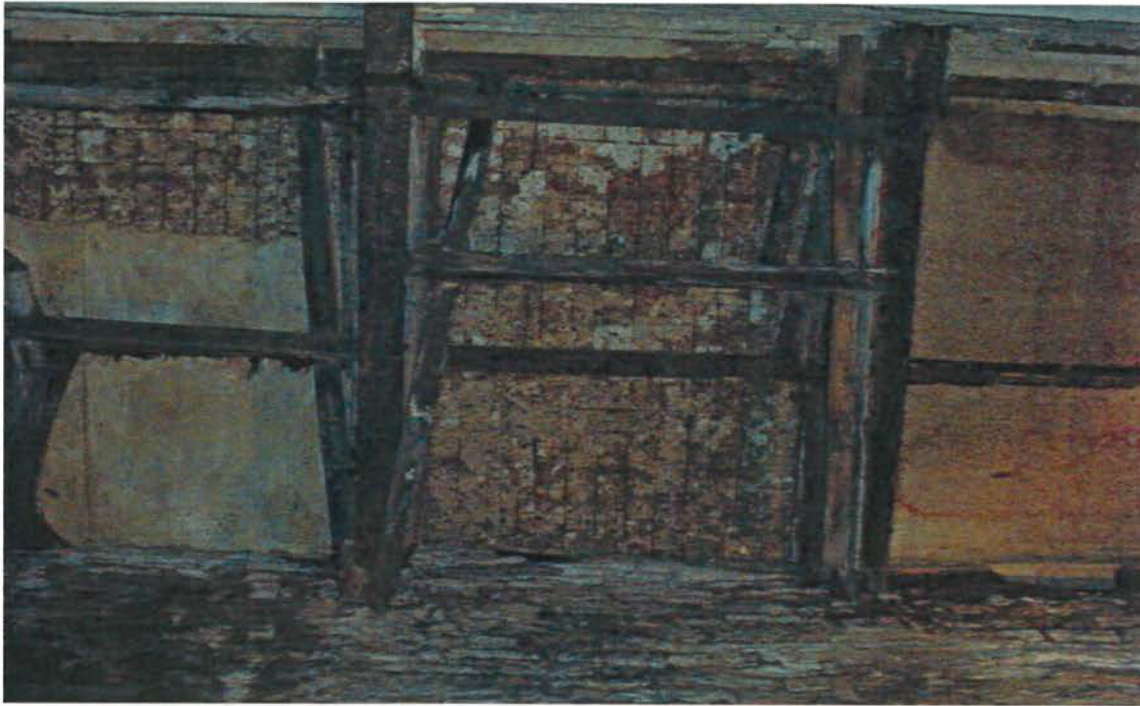
Image 5: (South Section) Close up of roof structure at south end.
