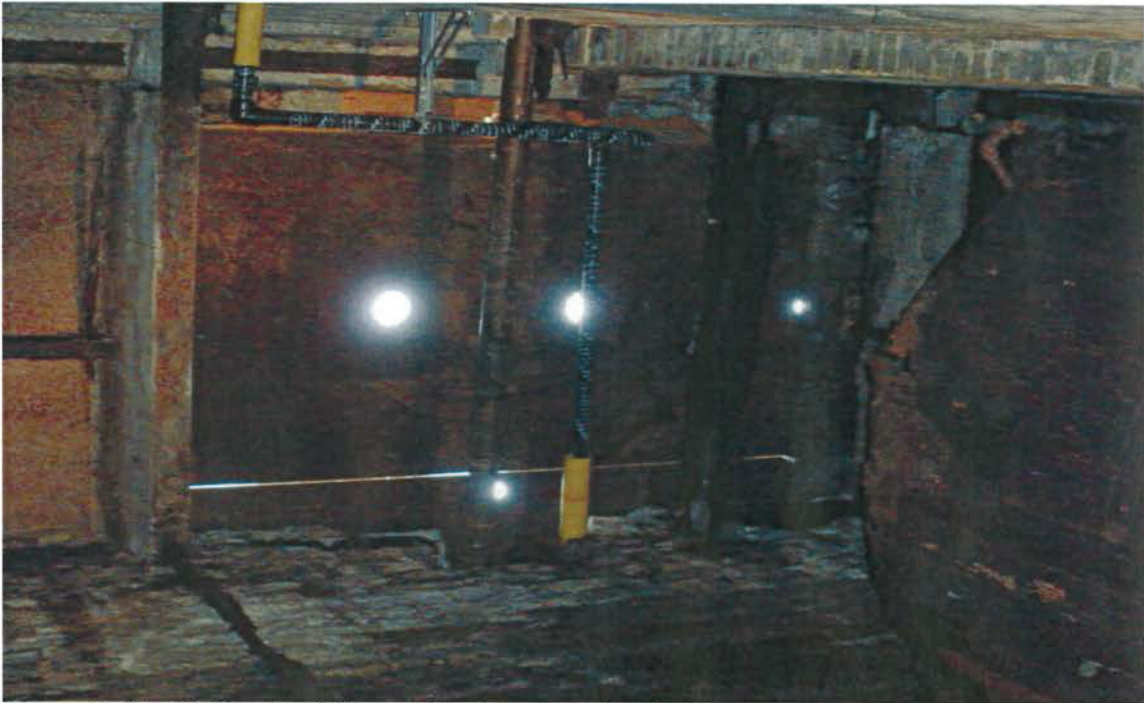
Image 8: (South Section) New natural gas service looking west.
