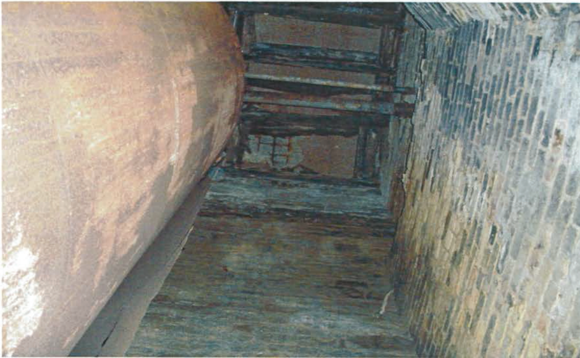
Image 2: (South Section) Roof structure at north end.
