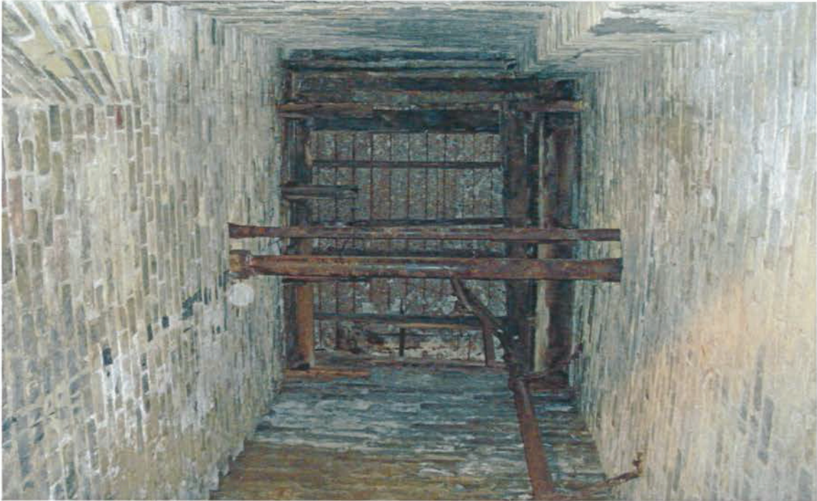
Image 17: (North Section) Roof structure.
