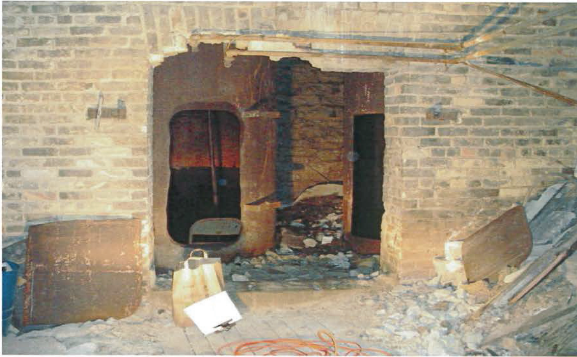
Image 1: (South Section) Opening in east wall.
