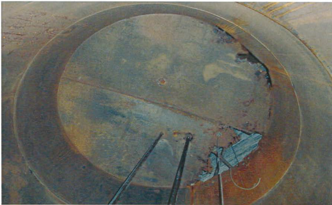
Image 16: (South Section) Roof of steel tank.
