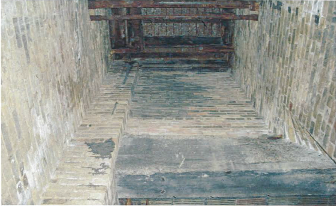
Image 18: (North Section) East wall.
