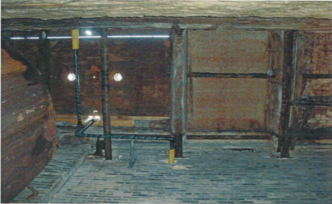
Image 7: (South Section) New natural gas service looking east.
