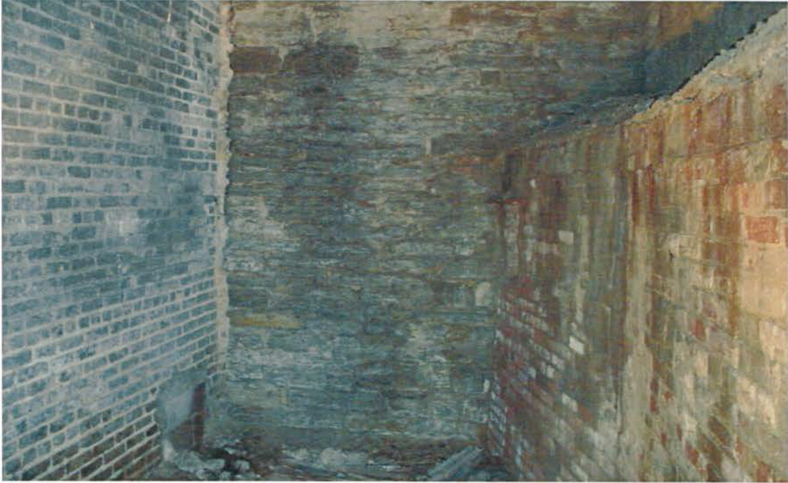
Image 10: (South Section) South wall. Angled wall on right.
