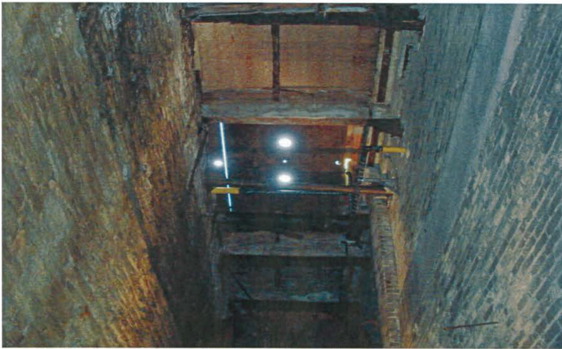
Image 6: (South Section) Roof structure looking north.
