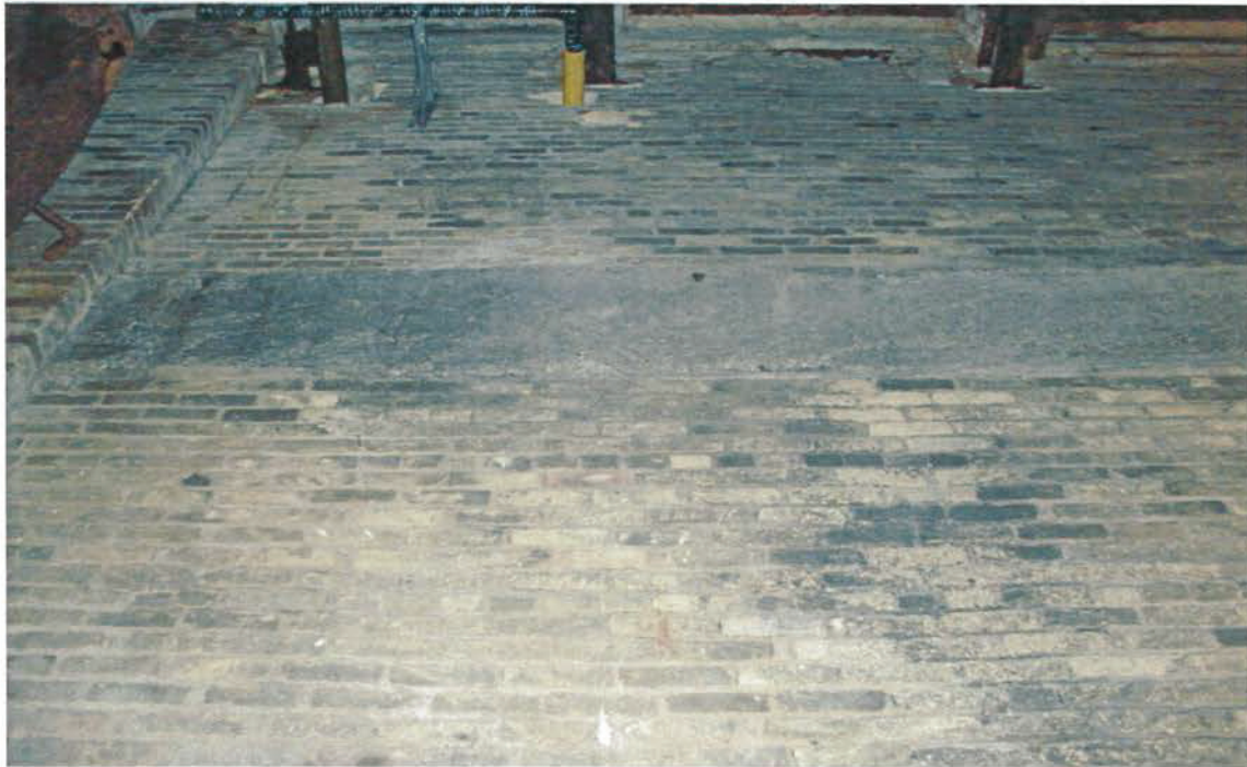
Image 12: (South Section) East wall.
