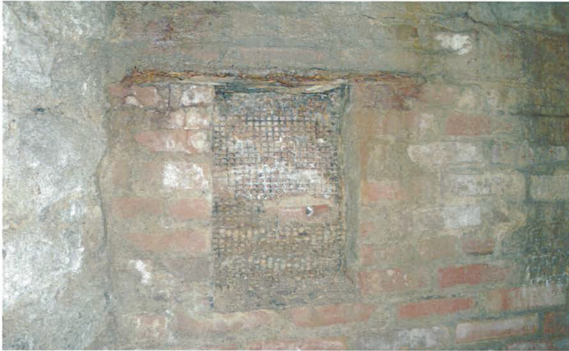
Image 11: (South Section) Opening in angled west wall.
