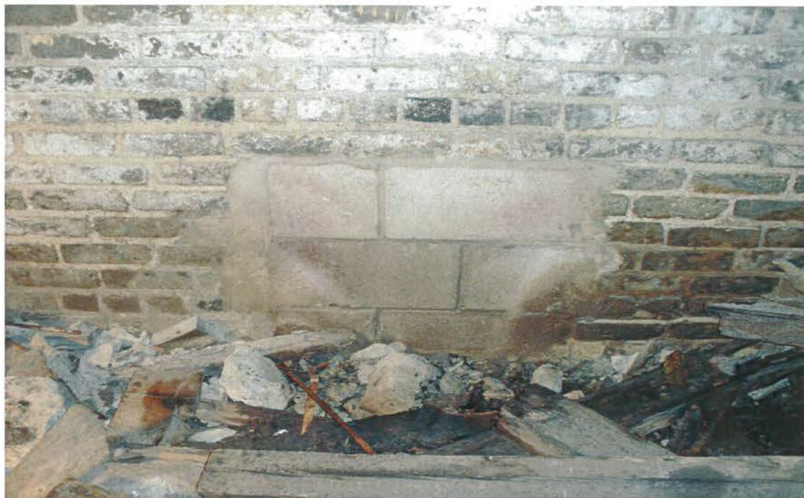
Image 13: (South Section) Block infill at east wall.
