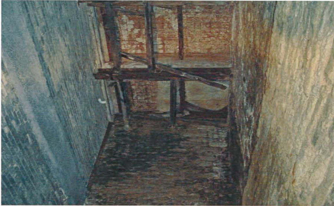
Image 3: (South Section) Roof structure at south end.
