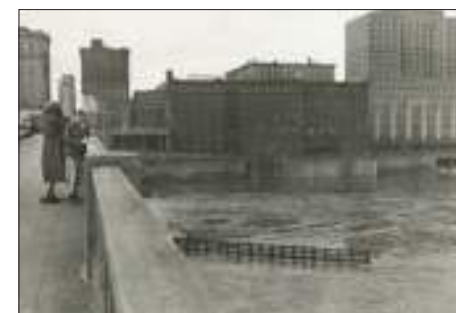
Figure 34. Bluff below Wabasha Street Bridge in ca. 1917 with cribbing (left); Corps of Engineers embankment, 1936, shown during 1951 flood (right).
