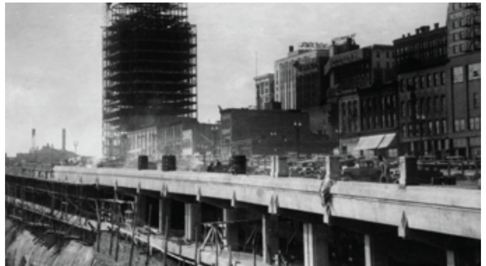
Figure 31. The skeleton of St. Paul City Hall/Ramsey County Courthouse rises above the new Kellogg Boulevard, ca. 1930.
