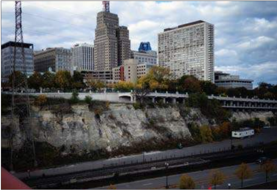
Figure 40. A portion of the project area viewshed from the Wabasha Bridge, September 2015.
