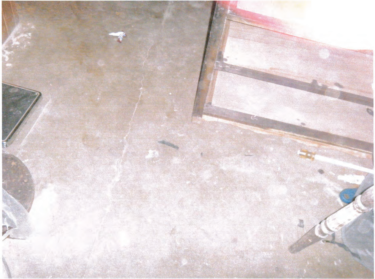
Photo taken 11/1/12 @ 12:37 p.m. - Down stairs
