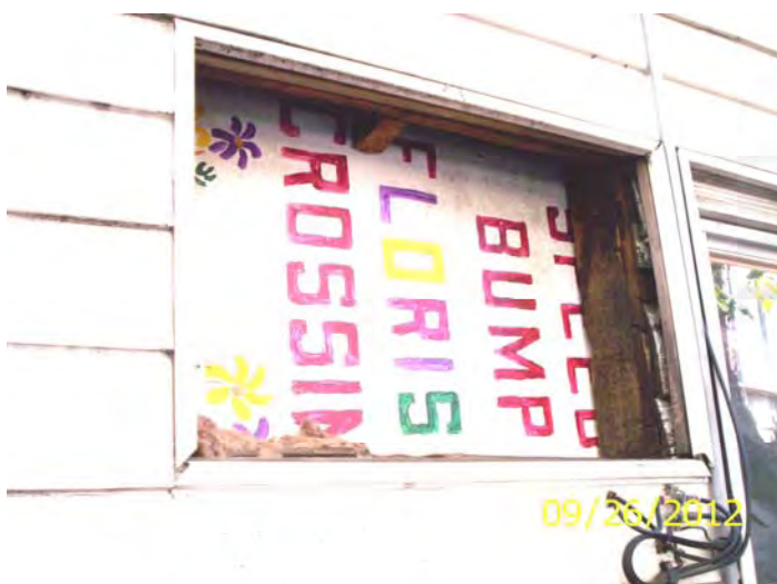
Opening in the north wall
