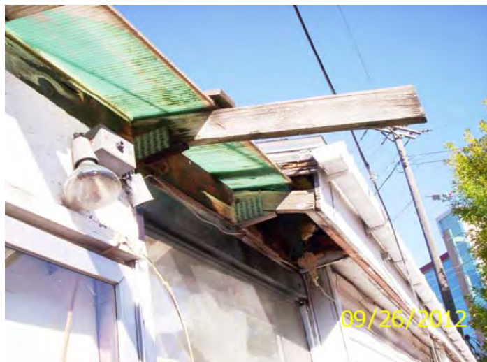
South side eave
