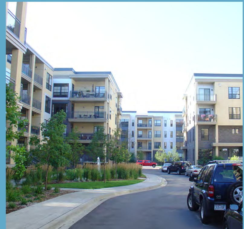
FIGURE 4.5 - Extending the existing highly successful pattern of residential development on Berry (pictured above) will help to increase the local population and support the expansion of local retail services.
