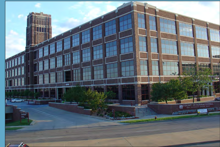
FIGURE 1.7 - Employment uses such as the Court International (above) and the University Enterprise Laboratories play an important role in supporting the Station Area as a place for people to both live and work.
