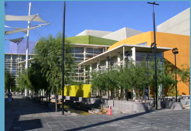
FIGURE 4.9 - Focusing office and employment uses around a plaza or open space system such as at this development in Arizona does not only help to create an address, but encourages employee interaction and fosters innovation.
