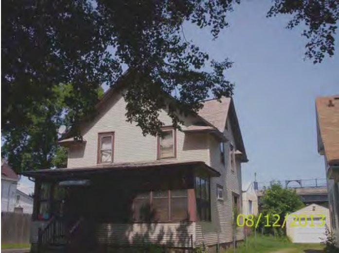
South and east sides, posting
