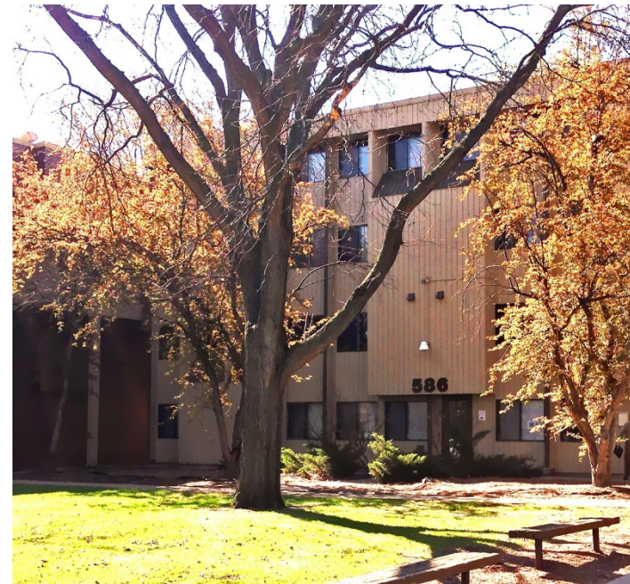
Jamestown Apartment Photo source: tchdc.org
