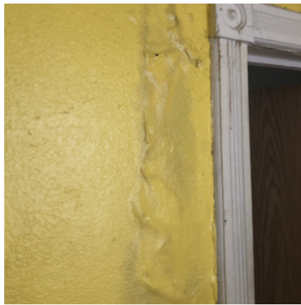
Living Room - Walls/Ceiling
