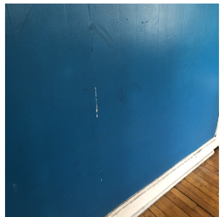
Living Room - Walls/Ceiling
