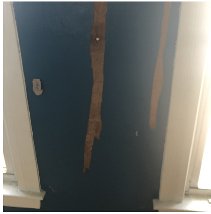
Living Room - Walls/Ceiling
