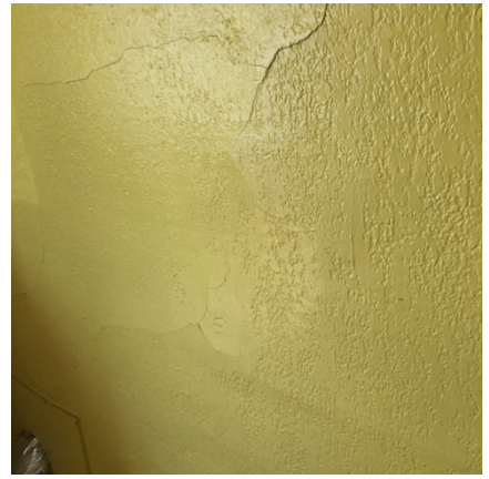
Living Room - Walls/Ceiling
