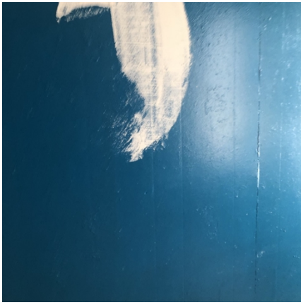
Living Room - Walls/Ceiling
