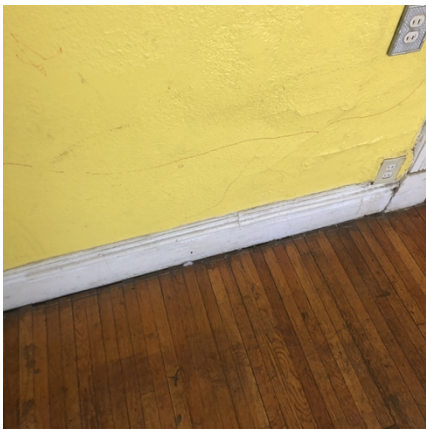
Living Room - Walls/Ceiling
