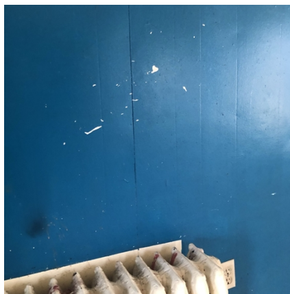
Living Room - Walls/Ceiling
