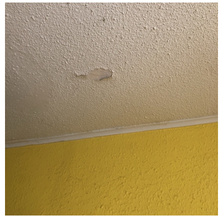
Living Room - Walls/Ceiling
