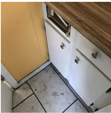
Kitchen - Cabinets/Counter Tops
