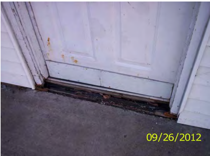
Front door threshold
