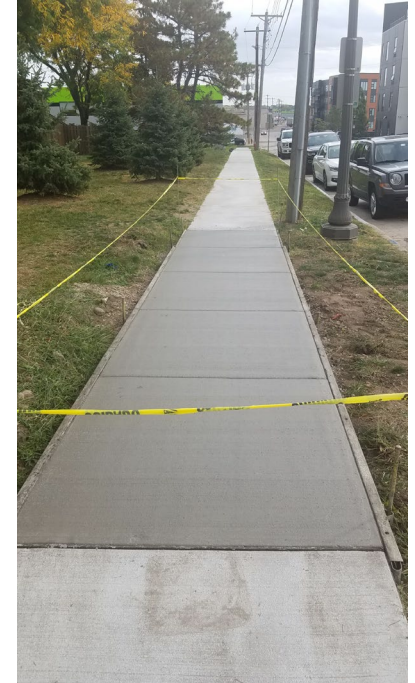
Pedestrian Infrastructure at Raymond and Seal Hi-Rise
