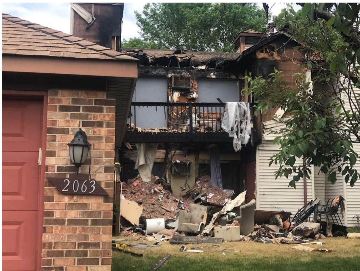
2063 Parkside Drive, Photos from 6-7-22
