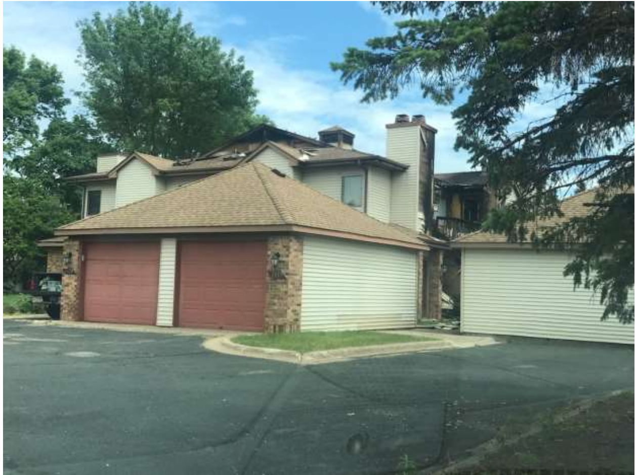
2063 Parkside Drive, Photos from 6-7-22
