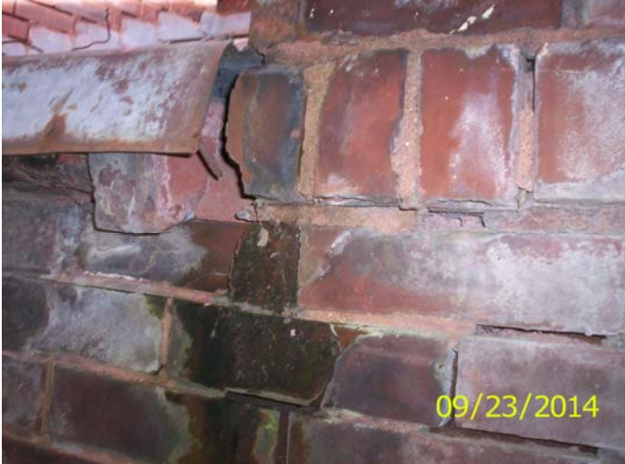
Deteriorated masonry
