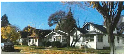
One and a half story single family dwellings on Snelling south of St. Clair Ave.
